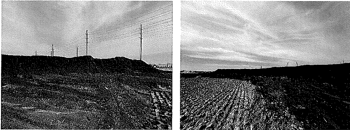
Figure 11: Foundry sand compiled on the Former Brook Park Ford Property. McBride Dale Clarion site evaluation photos, Photos Captured: 24 July 2026.
